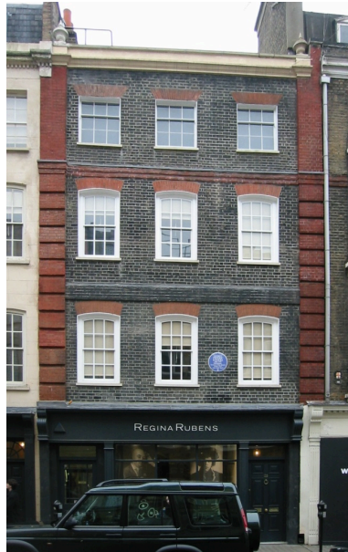
Figure 3. Handel House at 25 Brook Street, Mayfair, London
