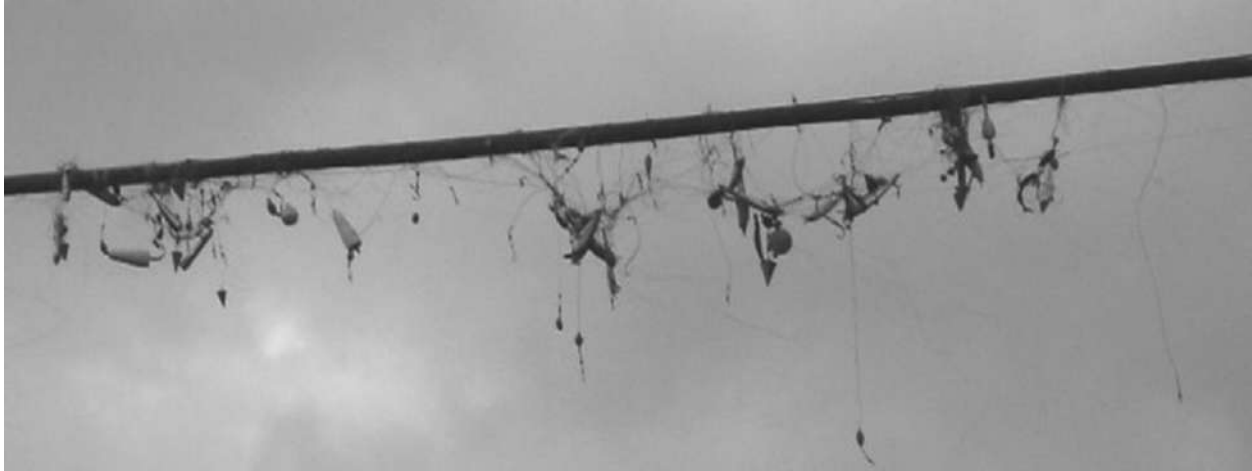
FIGURE 3-1 Fishing lines, weights, and lures caught in a power line. (Source: Authors)
