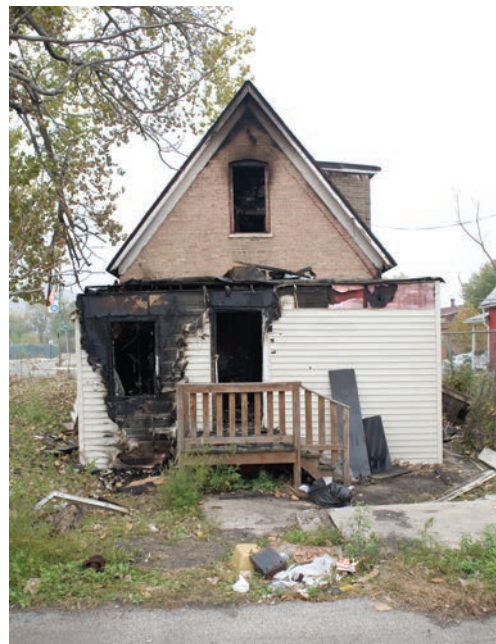
FIGURE 17-6 Typical V pattern illustrating upward movement of the fire.
