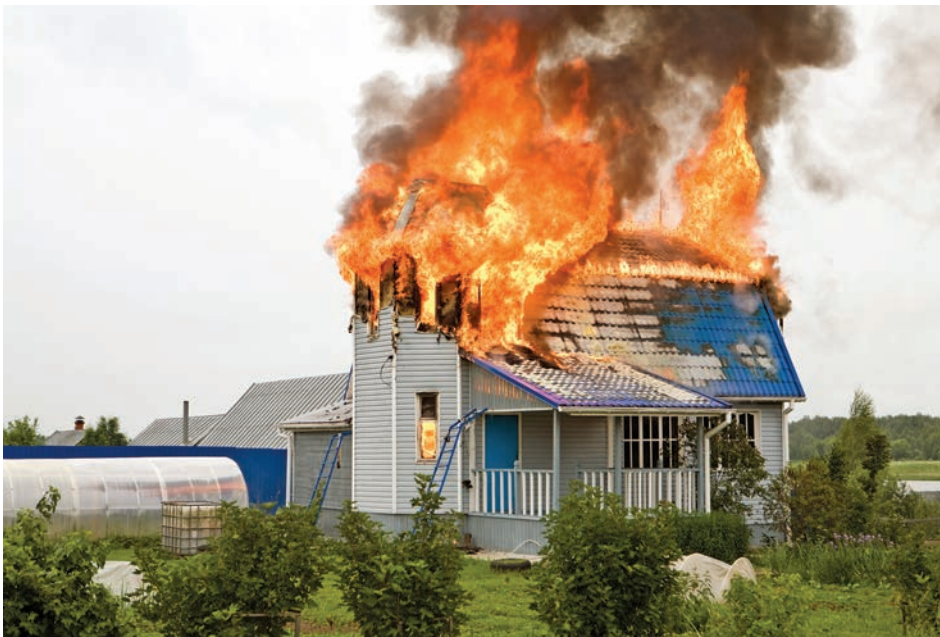
Convection causes flames to rise to the upper floor of a burning structure.
