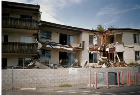
Figure 6.8: Northridge Meadows Apartment Building Collapse 34
