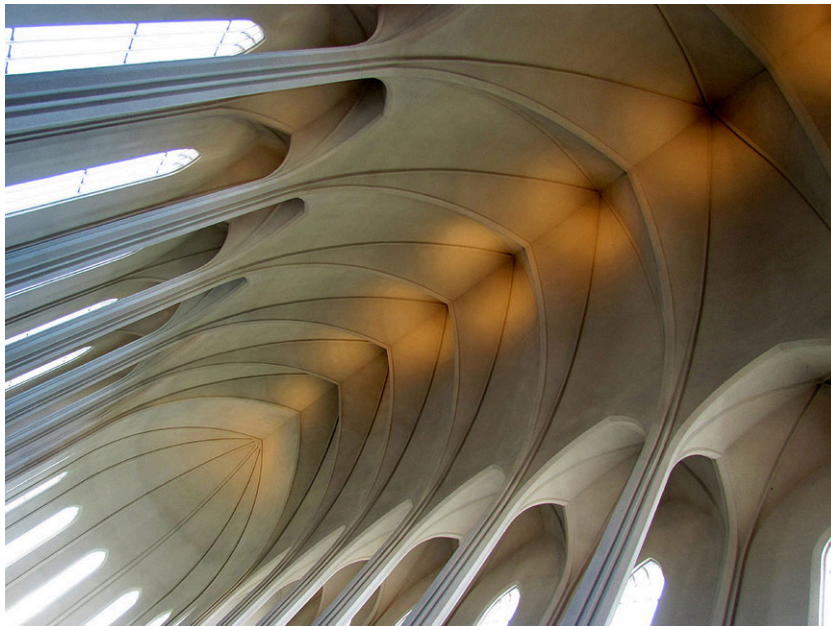
Figure 10.42 The appearance of triangles in buildings is part of modern-day architectural design. (credit: "Inside Hallgrímskirkja church, Reykjavik, Iceland" by O Palsson/Flickr, CC BY 2.0)
