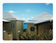
Bermuda has no fresh water other than falling rain, so roofs are designed to funnel rain down into underground holding tanks.
